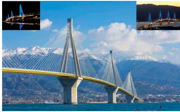
Figure 16. 2380 m Rio Antirrio fanned cable-stay bridge.
