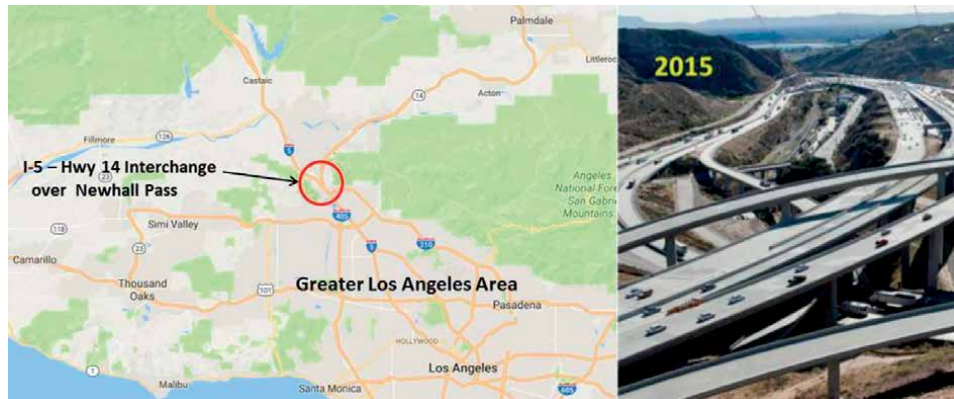
Figure 5. Interstate I-5 and State Road 14 interchange over the Newhall Pass.
