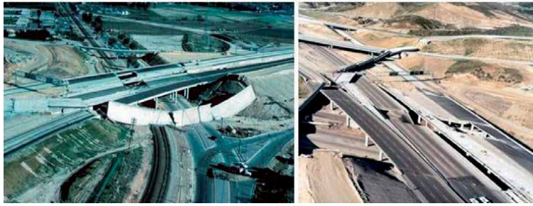
Figure 9. Failure of I-210 overpass to I-5 south.
