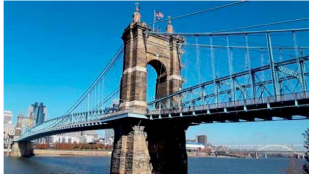
Figure 15. John A. Roebling Bridge Cincinnati OH.
