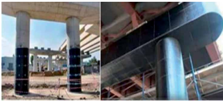
Figure 18. CFRP strengthening of bridge bents and columns.
