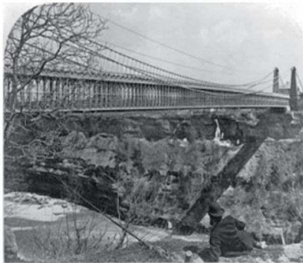
Figure 14. 822 ft Niagara railroad suspension bridge.
