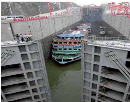
Figure 1. Vertically framed Miter dam.
