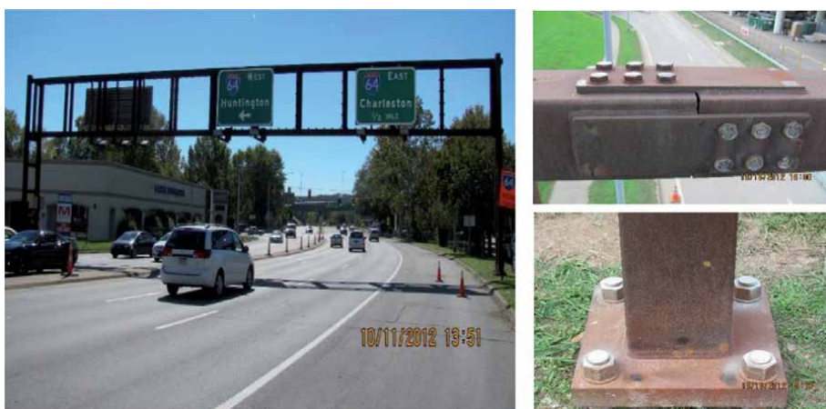
Figure 5. Dual-shoulder-mount-truss weathering-steel overhead sign structures.
