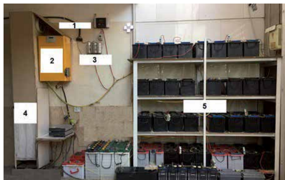
Figure 19. Detailed illustration of a 10 kW experimental rooftop off-grid solar system in Baghdad (Source: Dr. Jaafar Ali Kadhum Al-Anbari).
