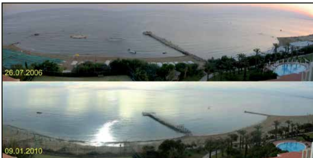
Fig. 12. Two panoramic views of the Perissia Hotel Beach at 26.07.2006 and 09.01.2010 showing the before and after remedial measures
