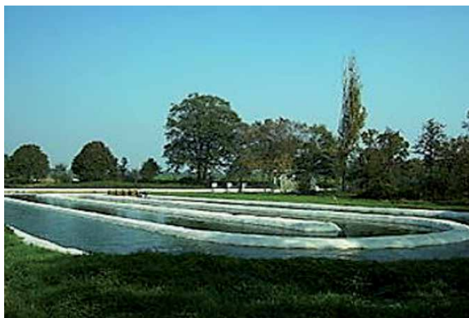
Figure 10. Algae raceway pond: The microalgae culture broth is constantly kept in motion with a powered paddle wheel [23].
