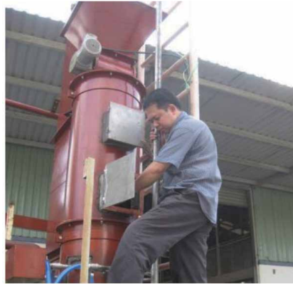
Figure 5. Fixing a downdraft gasifier after a bridging problem happened.
