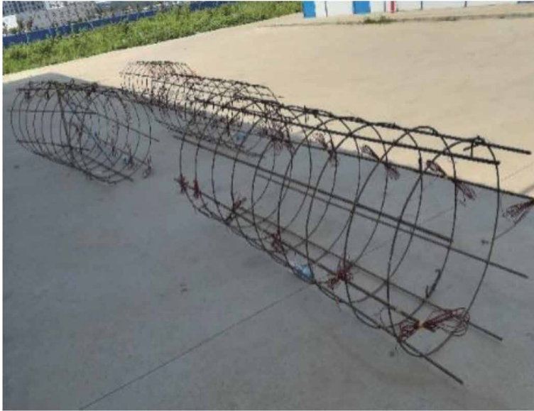
Figure 3. Steel reinforcement cage.
