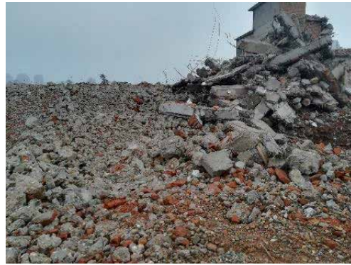
Figure 1. Demolition and transformation of DCLs.
