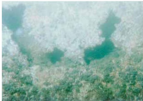
Fig. 1. An sample underwater photo taken during a pier inspection.
