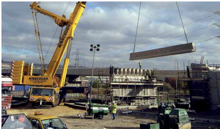
Figure 1. Precast girders with GRP deck panels for in situ deck.
