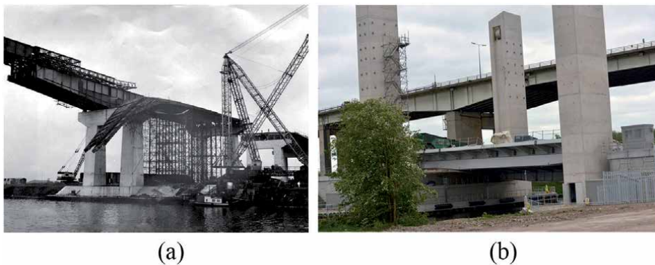
Figure 4. (a) Barton bridge scaffold collapse (1959) and (b) lifting failure of a modern bridge (2016) (figures reproduced from Refs. [3, 14]).
