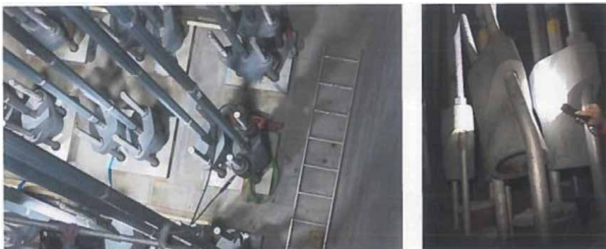
Figure 9. Hydrogen cracking in bolts (figure reproduced from Ref. [28]).
