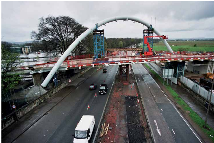
Figure 16. Temporary trestles near live highway.
