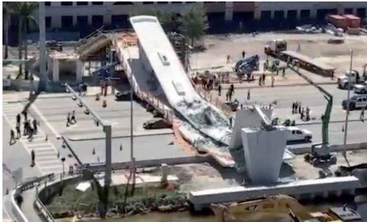
Figure 11. Florida Bridge collapse, 2019 (reproduced from Ref. [25]).
