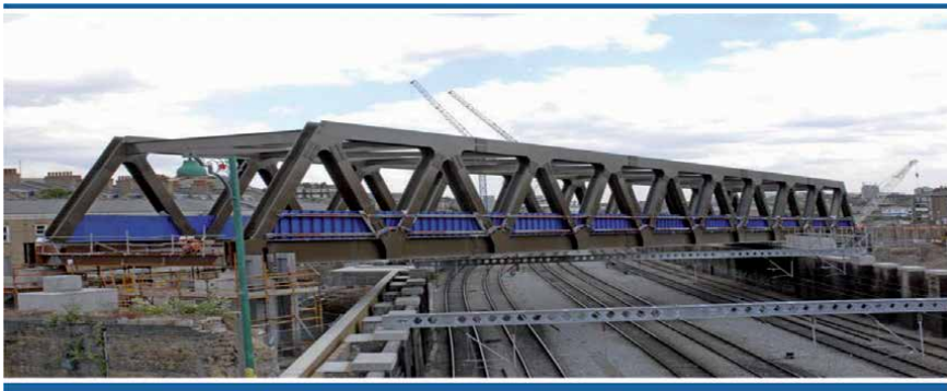
Figure 6. Bridge launch over railway (reproduced from Ref. [25]).
