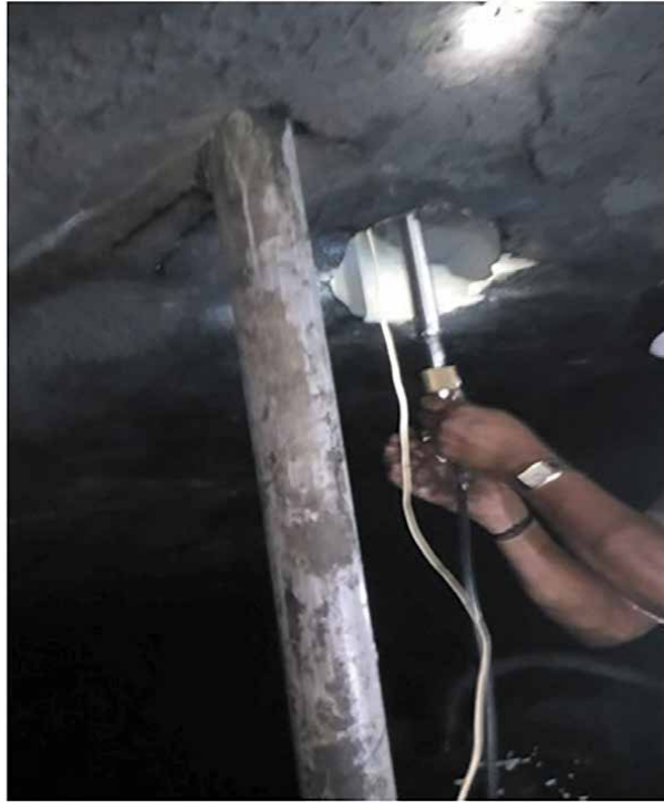
Figure 28. Installation of CISRO HI cell.
