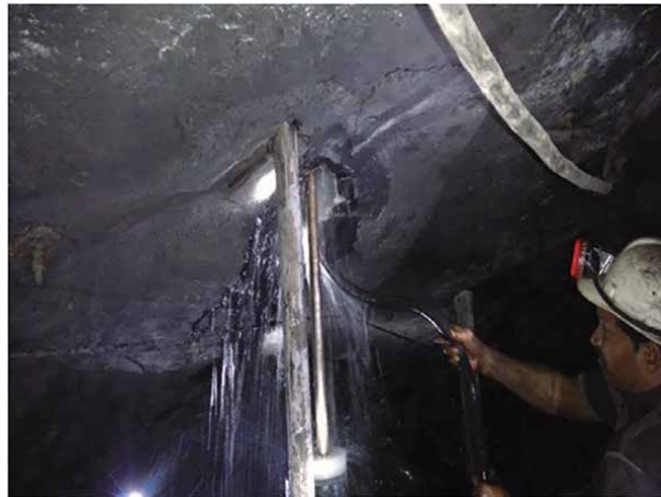
Figure 24. Drilling of EX size borehole (Pilot hole).
